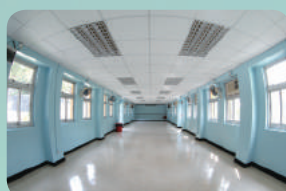
Renovation works at Tung Tsz Scout Centre
