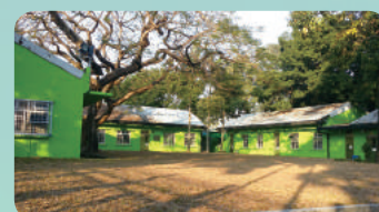
Painting works to building facilities of Choi Chee Ming Luen Kwong Scout Centre
