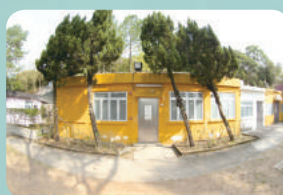
Window replacement works for Tung Tsz Scout Centre
