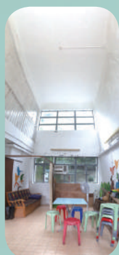
Concrete repair to Administration Building of Tai Tam Scout Centre
